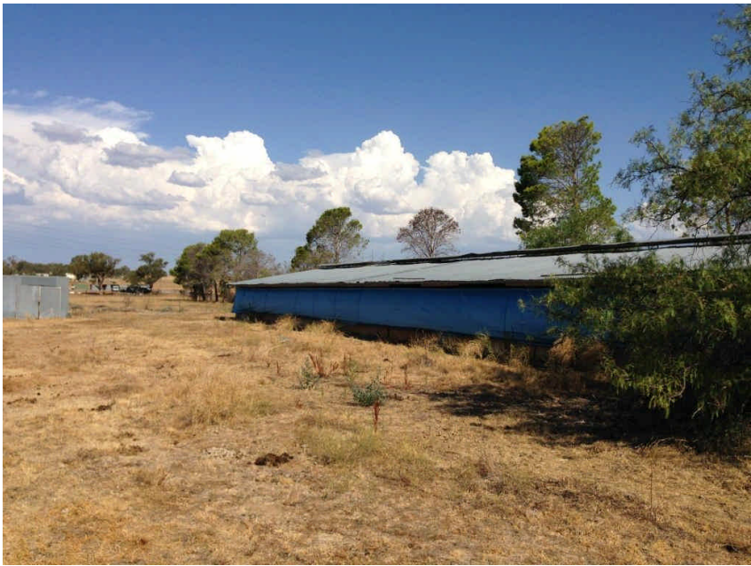
Plate 18: View of Disused Chicken Shed Lot 3 DP 38808
