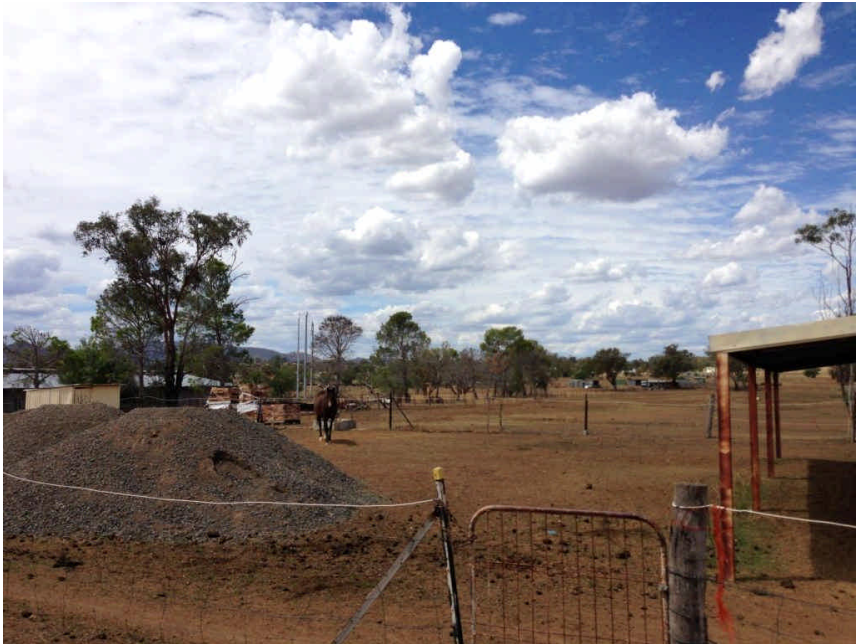
Plate 13: Gravel Stockpiled within Lot 2 in DP 38808
